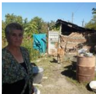
100% Repaid Liana Cattle – repair cattle shed Georgia
